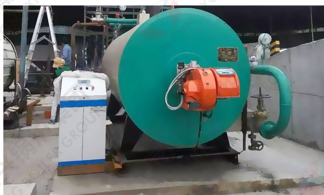
2015.04 广东广州长大公路工程160万大卡导热油锅炉 2015.04 1.6mkcal/h thermal oil boiler in Canton Changda Road Engineering Co.,Ltd
