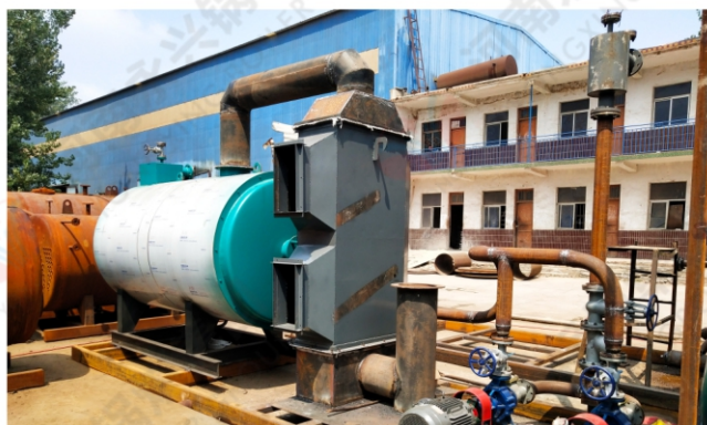
2016.10 浙江温州大和人造革厂80万大卡导热油锅炉 2016.10 0.8mkcal/h thermal oil boiler in Wenzhou Dahe artificial leather factory
